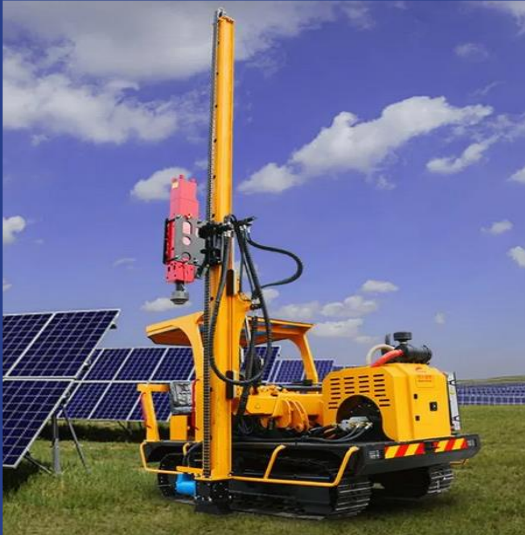
2 X PV Solar Farm Pile Driver Machine with Hydraulic Impact Hammer
